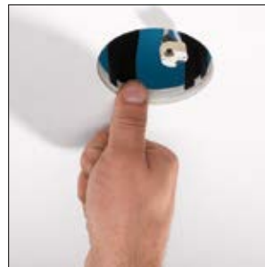
3. Push the spikes into the plasterboard to prevent shifting.
