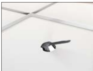
1. Insert the mounting support through the fixing hole.
